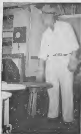
C. D. Goedgraz, assistant operator at the loading pumphouse, checks the gauge of the new fuel oil pump (pump is inside building). This operator is one of four who deals directly with tanker loading.
